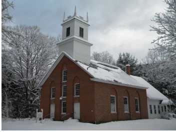
Brookline Meetinghouse Town Office location
